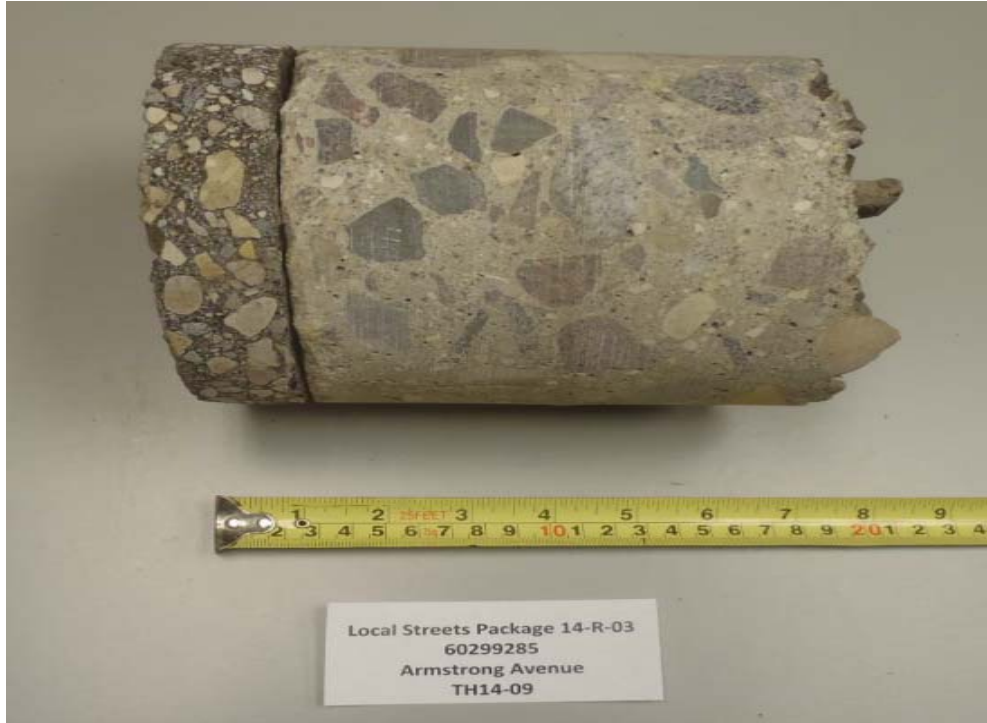
Photograph 5. Armstrong Avenue – TH14-09
