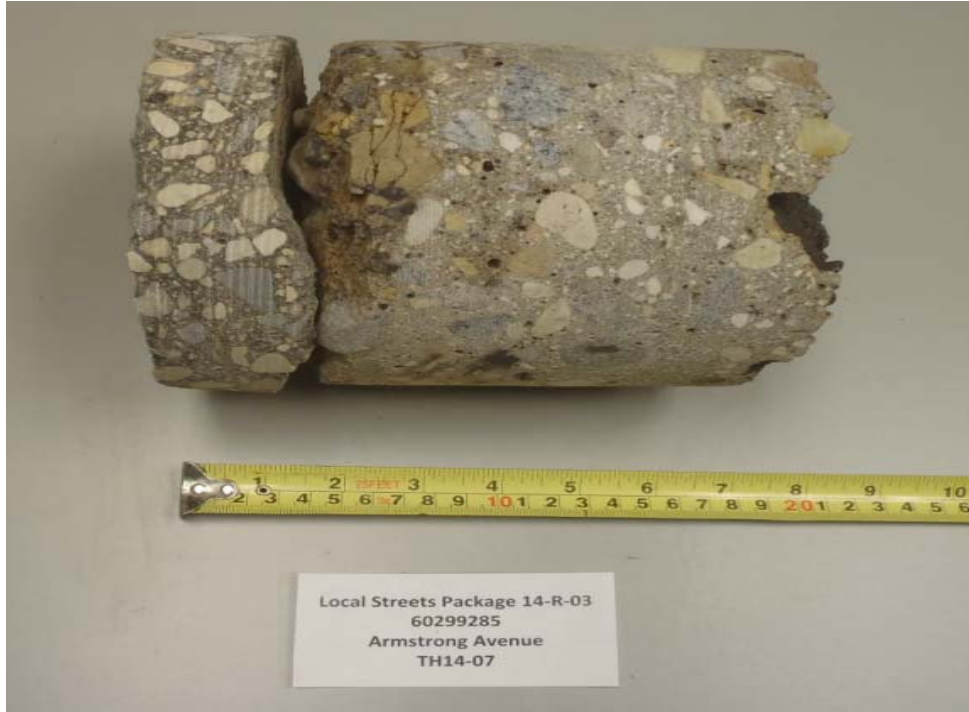
Photograph 3. Armstrong Avenue – TH14-07
